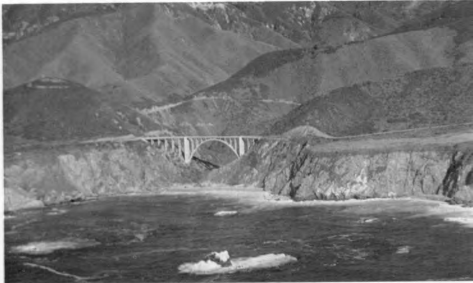
Bixby Creek Bridge, affectionately known as Rainbow Bridge, the longest single arch concrete span in the world. It is one of thirty three bridges connecting the Big Sur Highway.
