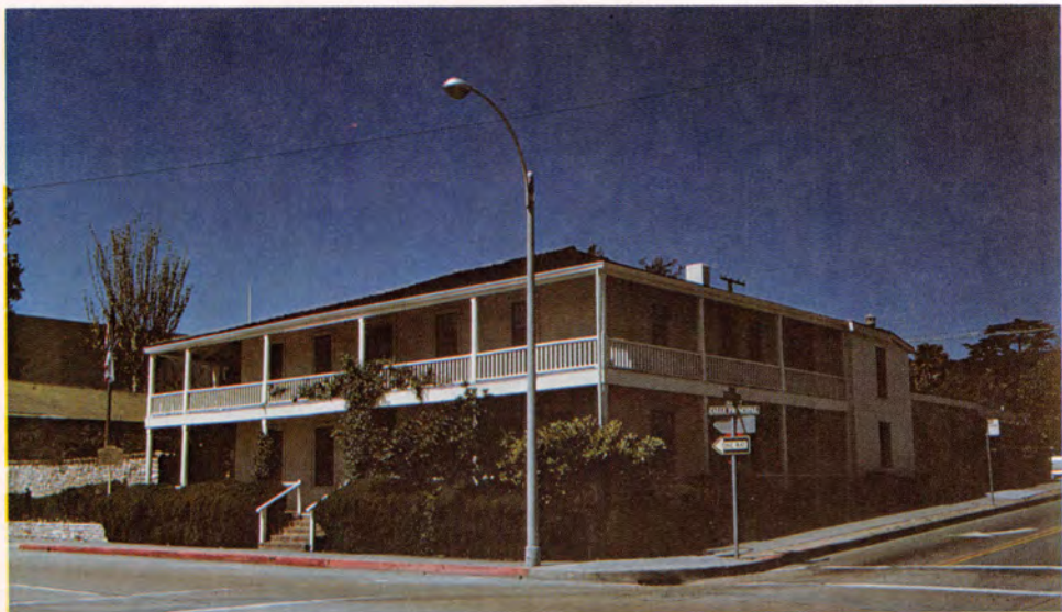
Larkin House, home of California's first millionaire. Note the hipped roof and encircling balcony. This house is a fine example of what became known as Monterey Colonial architecture.
