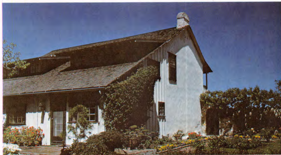
The Old Whaling Station. Note the wooden leanto. Many of the early adobes have wooden leantos added on to them. It was a simple way to provide space for kitchens and bathrooms, when people began including these rooms in the main house.
