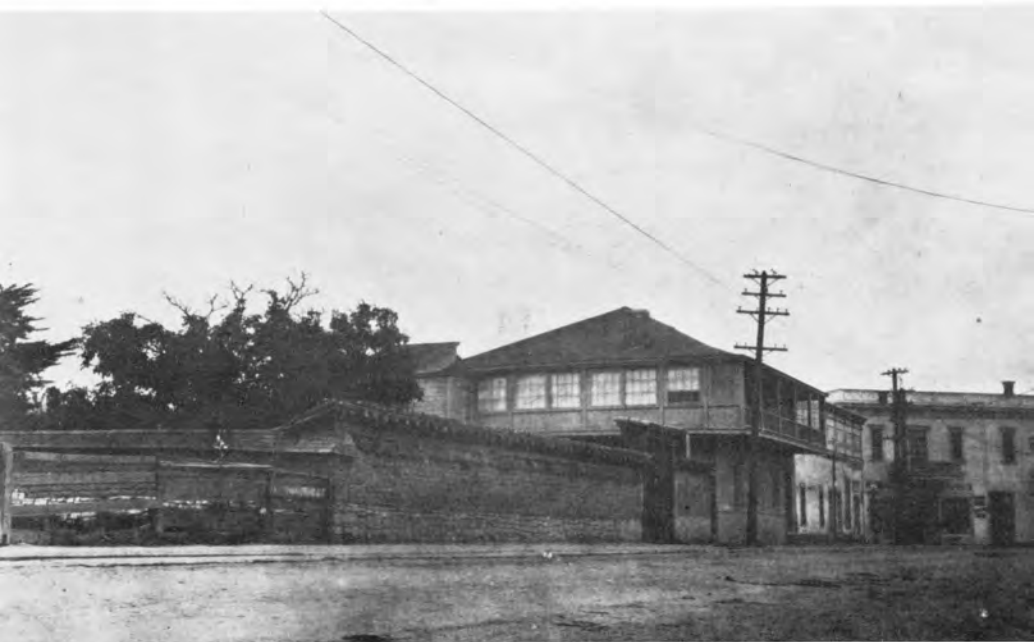
The Cooper House, home of John Rogers Cooper, fiery Yankee skipper. The adobe wall is in excellent condition. Close examination reveals the various things ... twigs ... straw ... plants that were mixed with the mud as a binder. No. 10
