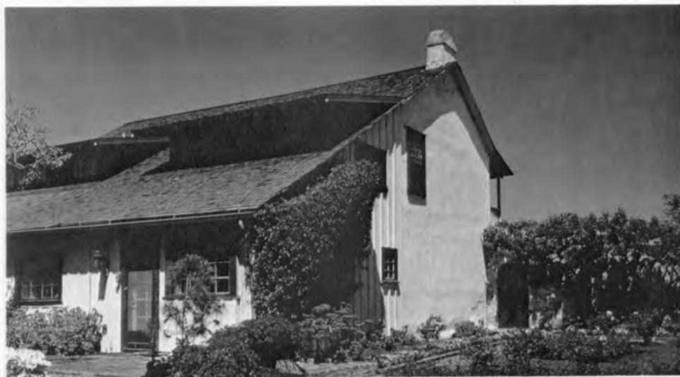
The Old Whaling Station. Note the wooden leanto. Many of the early adobes have wooden leantos added on to them. It was a simple way to provide space for kitchens and bathrooms, when people began including these rooms in the main house.
