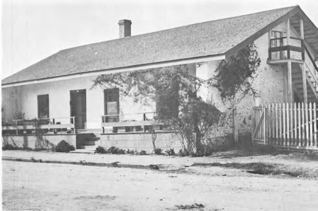
Casa Serrano, open on weekends 2-4 p.m. houses an excellent collection of early California furniture. The upper floor is reached by an outside stairway. Such stairs became known as "elopment stairs." Building property of Monterey History and Art Association. No. 23.
