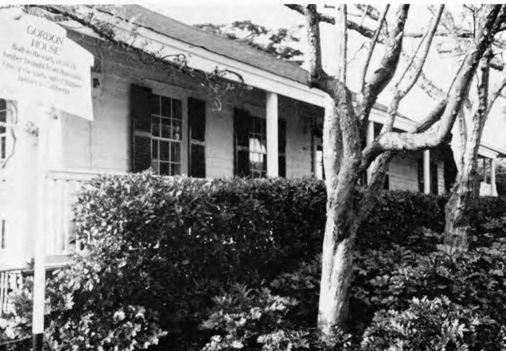
Gorden House, one of California's first houses built of wood. The lumber was milled in Australia, shipped to England, then reshipped around Cape Horn to Monterey. No. 18.
