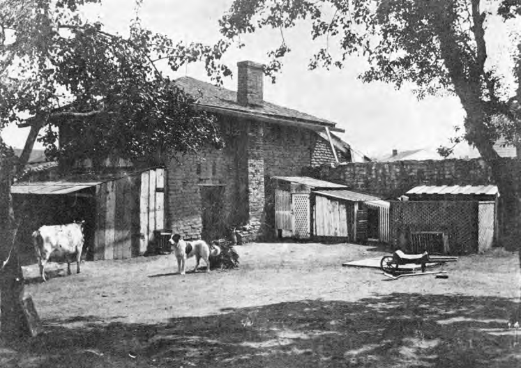
Early photo of House of Four Winds taken from the rear.
