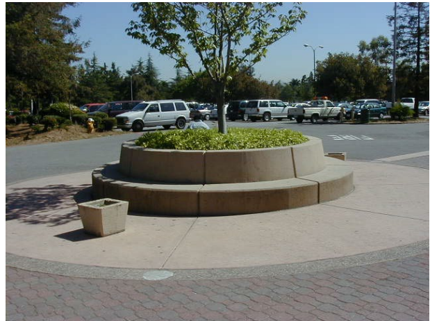
Do not post on benches/seating areas (things can get torn off causing litter)
