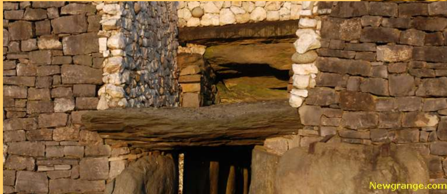
The Roofbox over the entrance where the solstice sun is beamed to the chamber.
